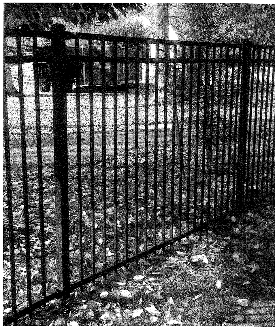
FENCE DETAIL PROPOSED FENCE TO MATCH EXISTING VERTICAL PICKET FENCE ON SITE (AS SHOWN ABOVE).
