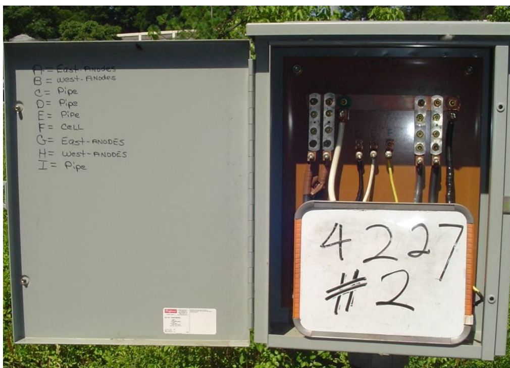
Figure 233 - Test Station 4227-2 close-up
