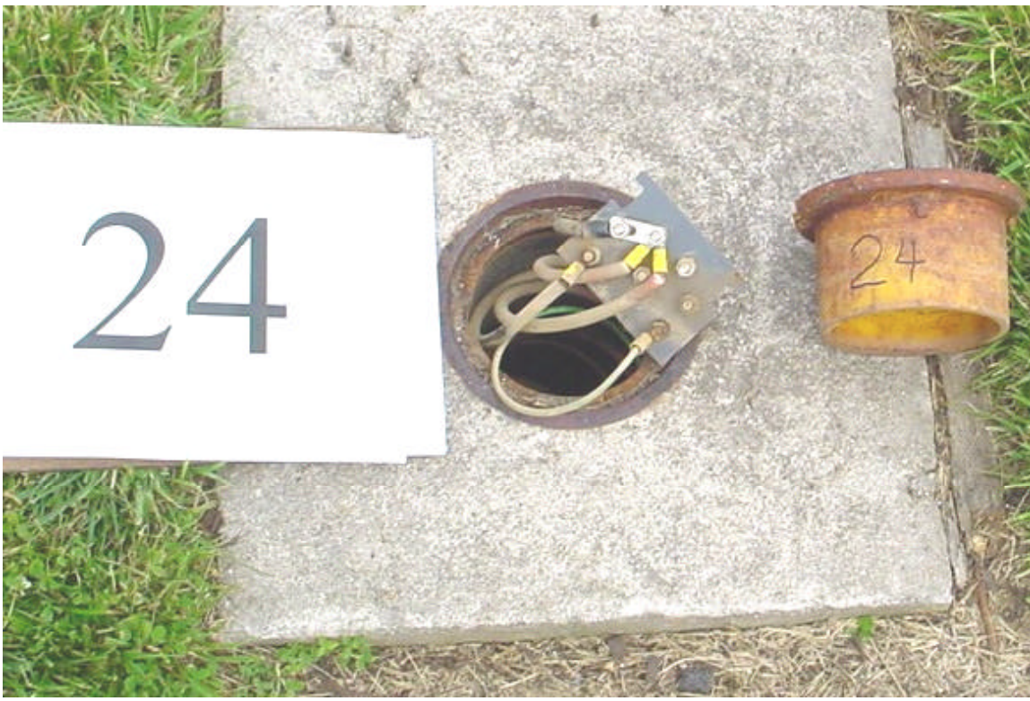
Figure 47 - Test Station #24, close-up
