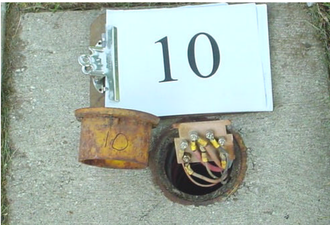
Figure 27 - Test Station #10, close-up
