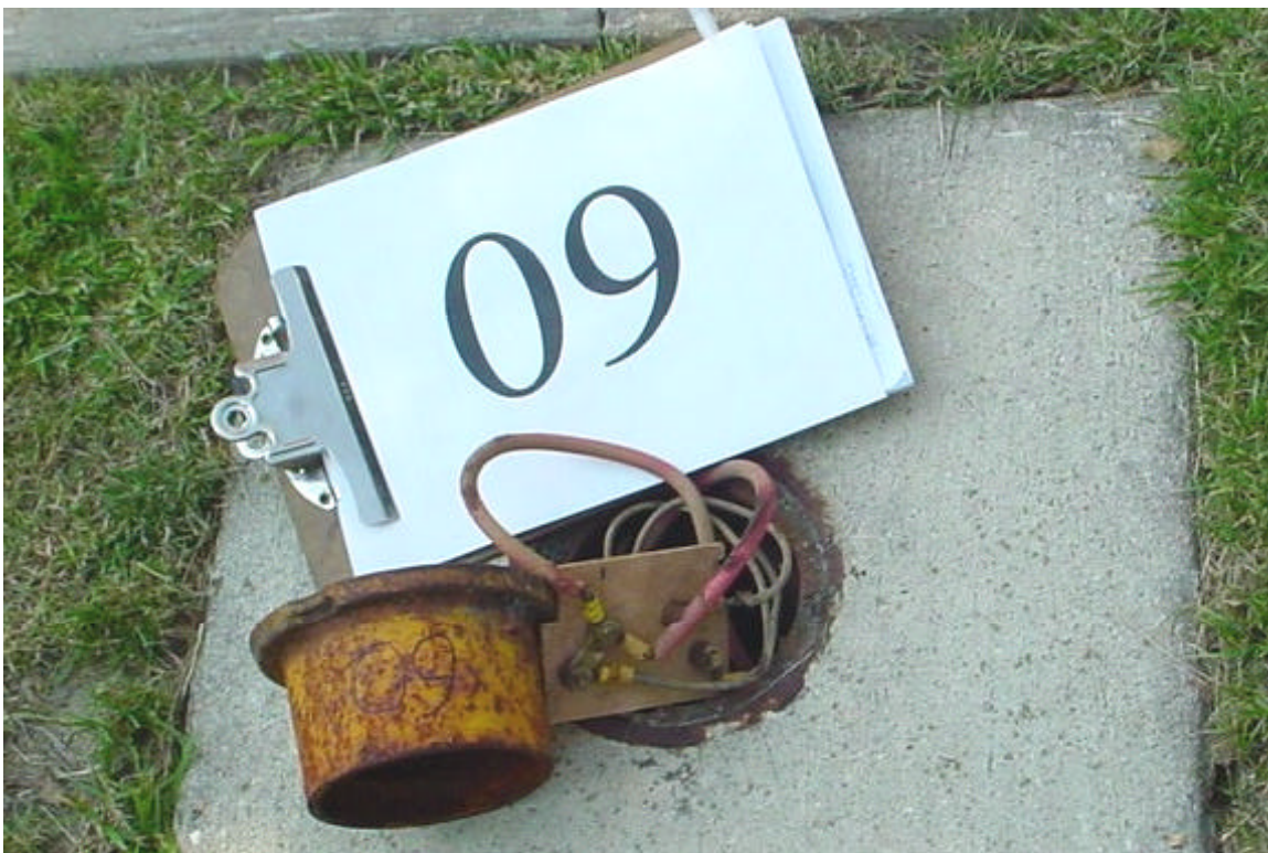
Figure 25 - Test Station #9, close-up
