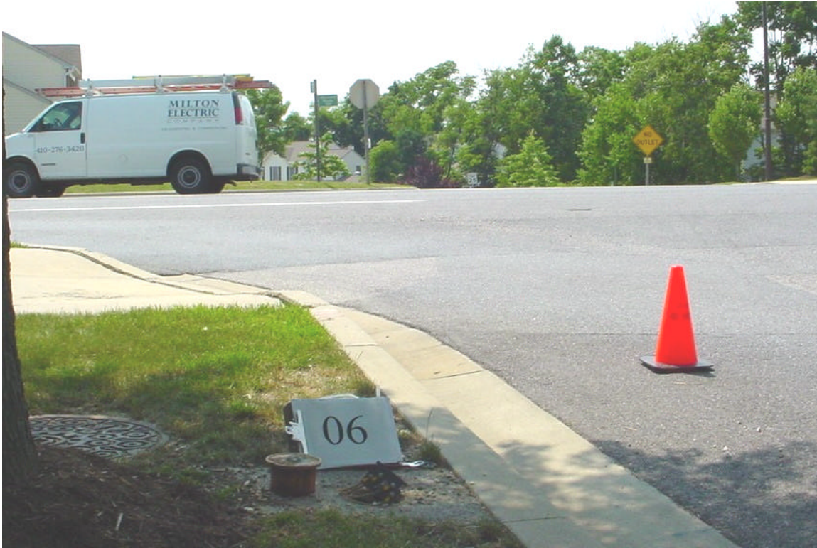
Figure 18 - Test Station #6, Old Stockbridge Drive & Route 108
