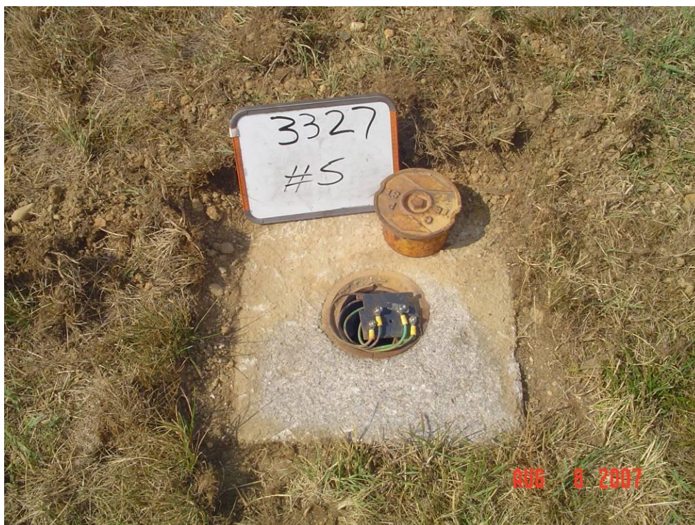
Figure 130 – Test Station 5 close up
