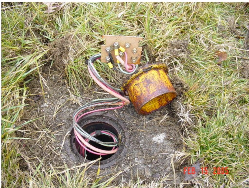
Figure 134 – Test Station 4 close up
