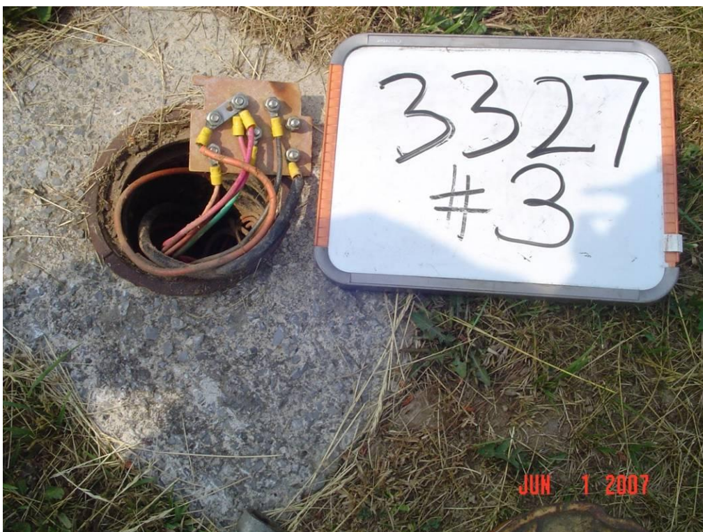
Figure 126 – Test Station 3 close up
