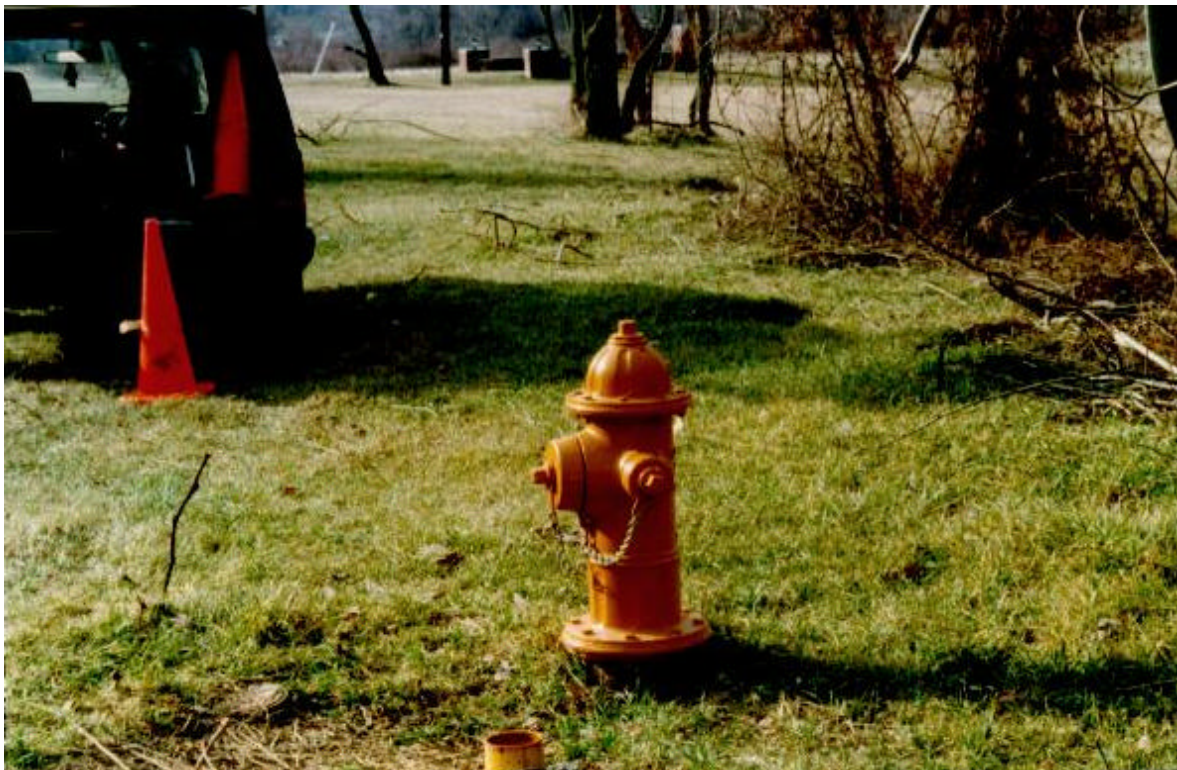
Figure D - 7. Test Station No. 04
