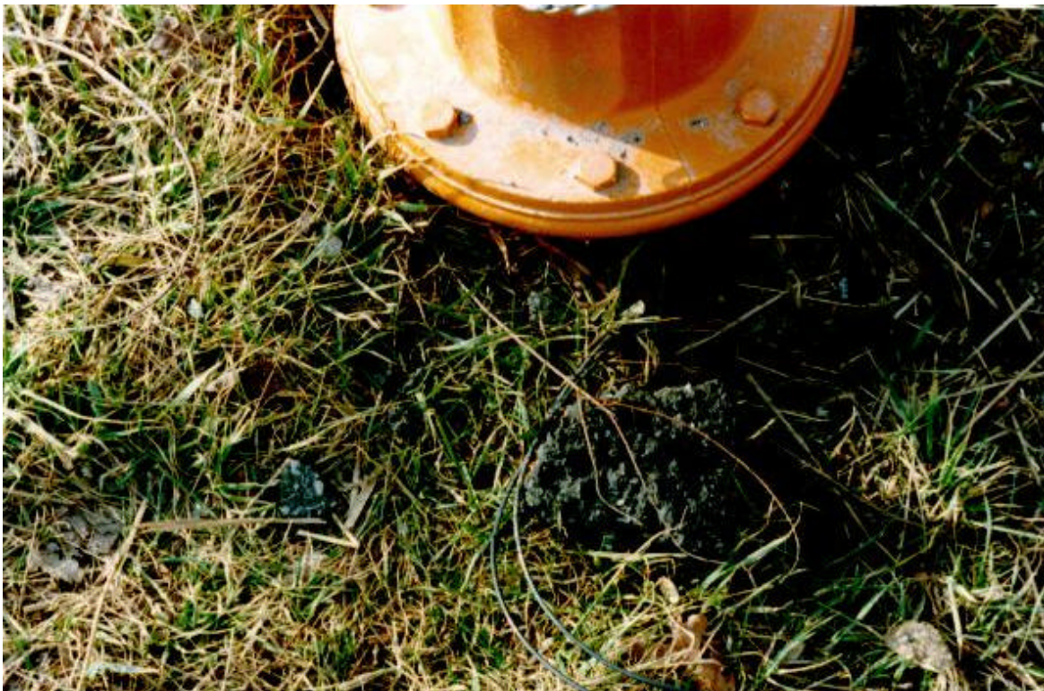
Figure D - 2. Close-up of Test Station No. 01
