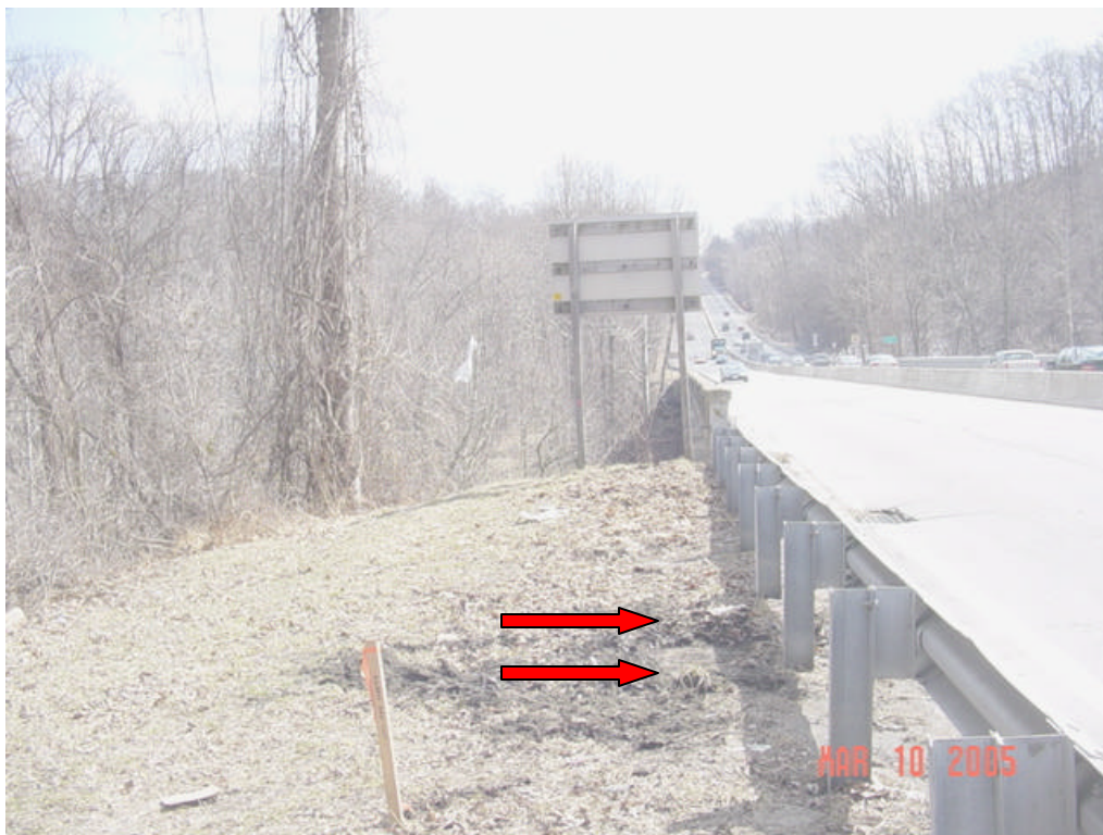
Figure 71 - Location of Test Stations on contract 8W
