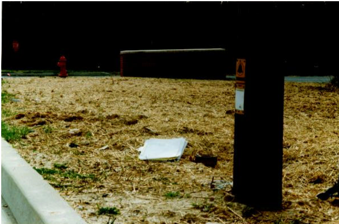
Figure C - 1. Test Station at Station Number 87+50
