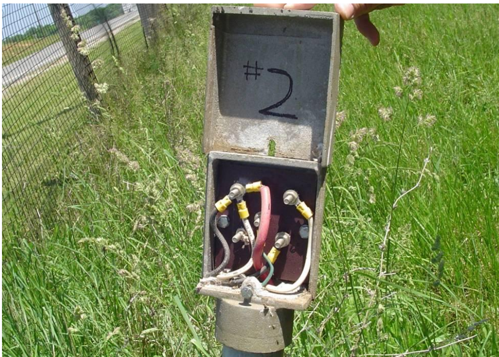
Figure 224 - Location of Test Station 2 at Alpha Ridge Landfill close-up
