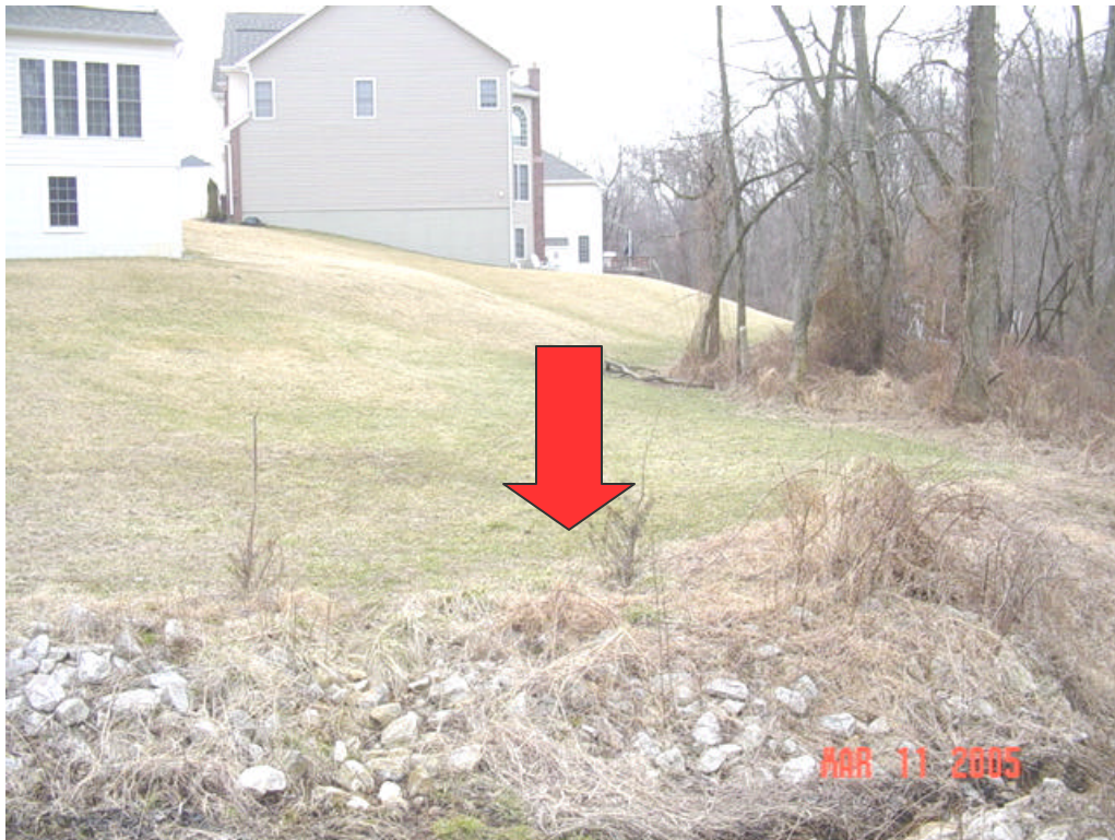
Figure 6 – General area of Test Station 8WM1 – Not Found
