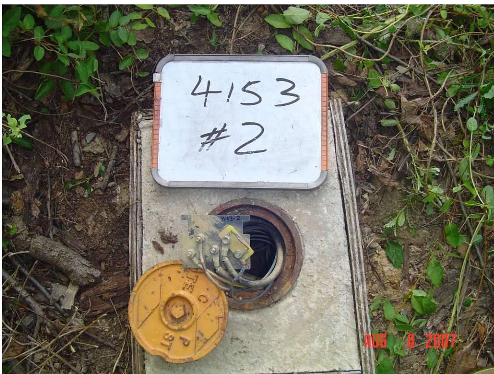
Figure 51 - Test Station 4153-2 close-up
