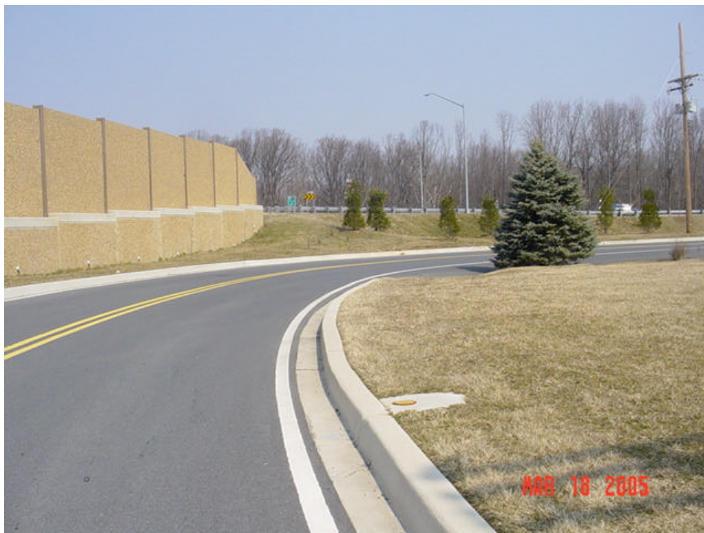
Figure 104 – Location of Test Station 9 - Hammond Parkway
