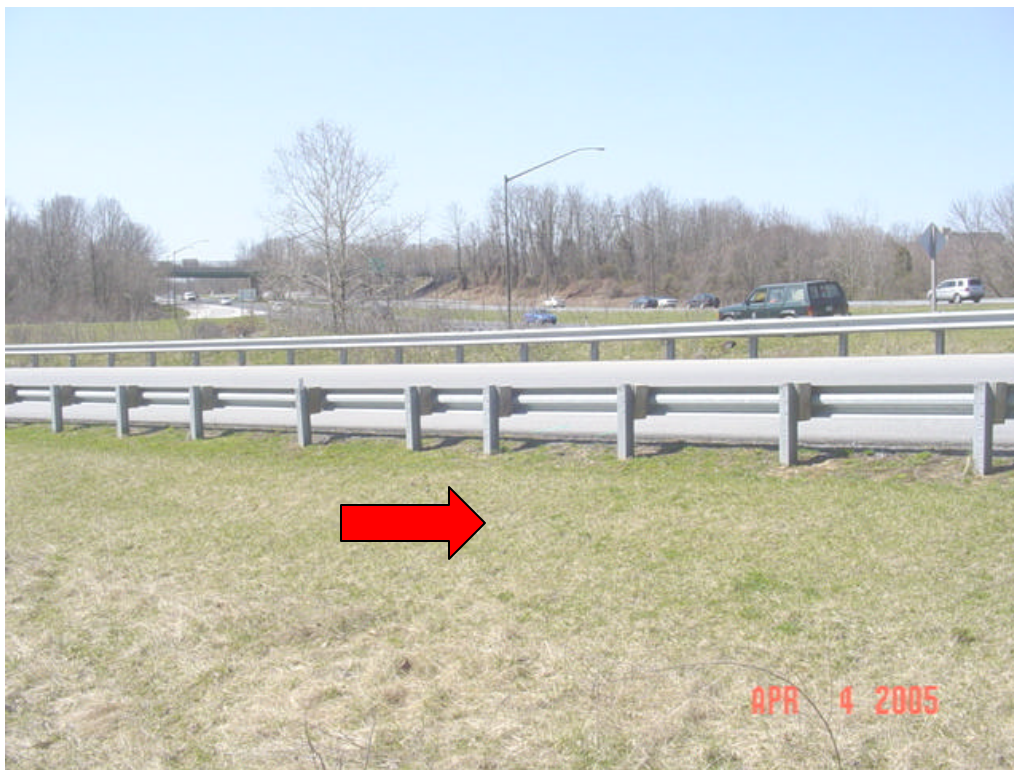
Figure 78 – General area of Test Station 3844-2 – Not Found
