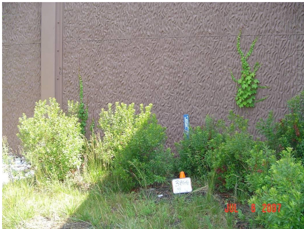
Figure 63 – General area of Test Station 3844-1 – Not Found
