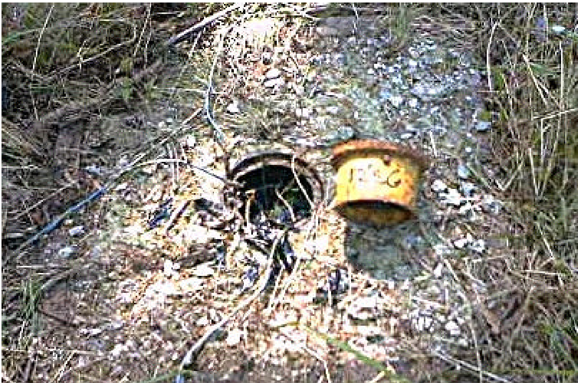
Figure 38 - Test station 12GS6, close-up
