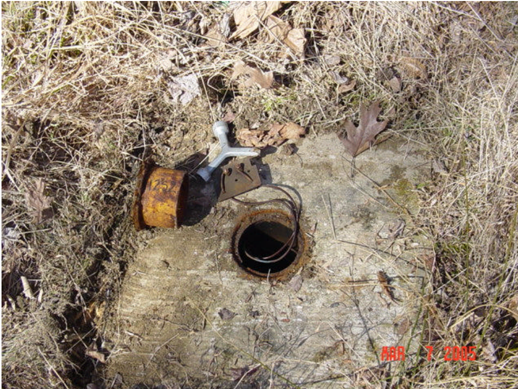
Figure 12 - Test Station 12GS2 close-up
