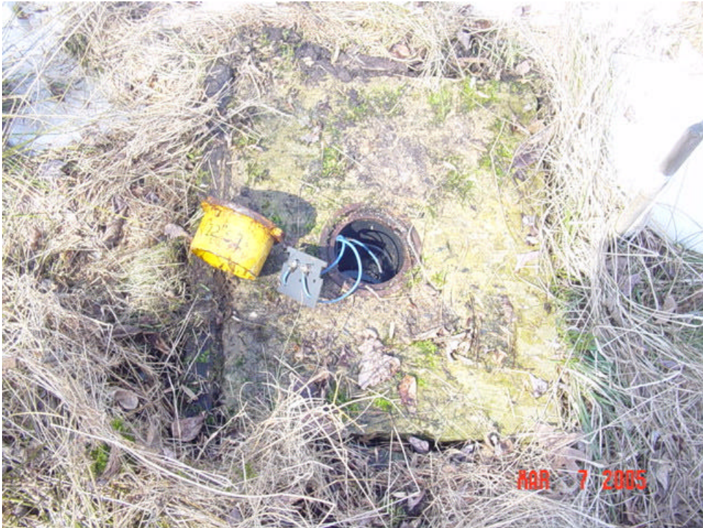
Figure 10 - Test Station 12GS1 close-up
