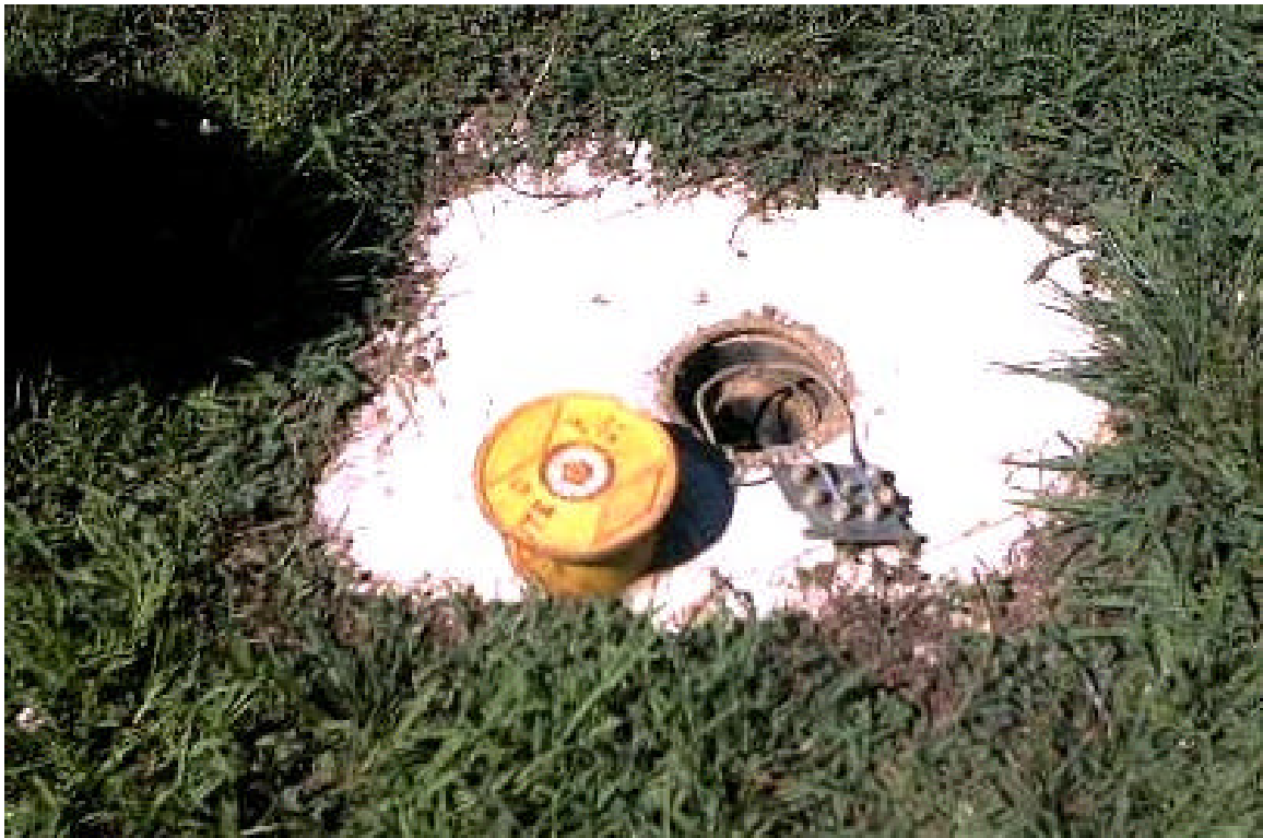
Figure 14 - Test station 12FM1, close-up
