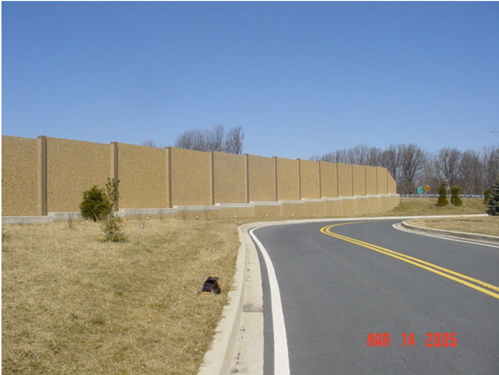
Figure 114 – Stray Current Test location site 1
