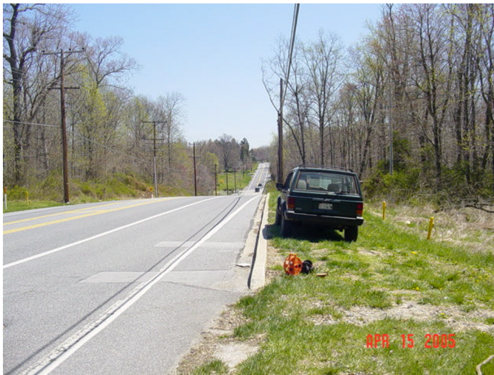
Figure 241 - Stray Current Test Location for contract 3479
