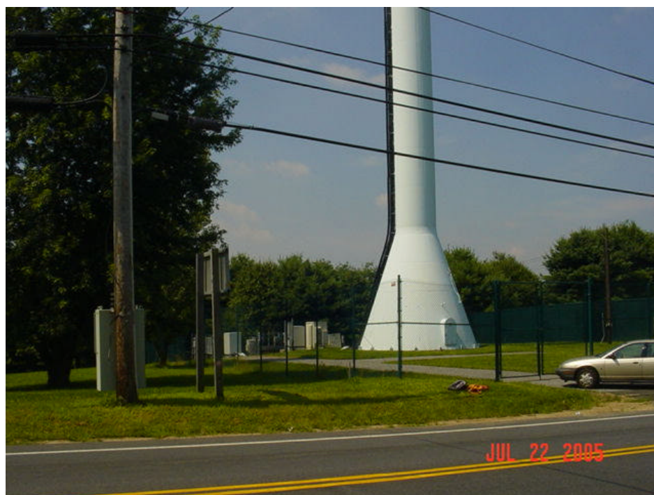
Figure 117 – Measuring stray currents near Bethany Lane and Route 99
