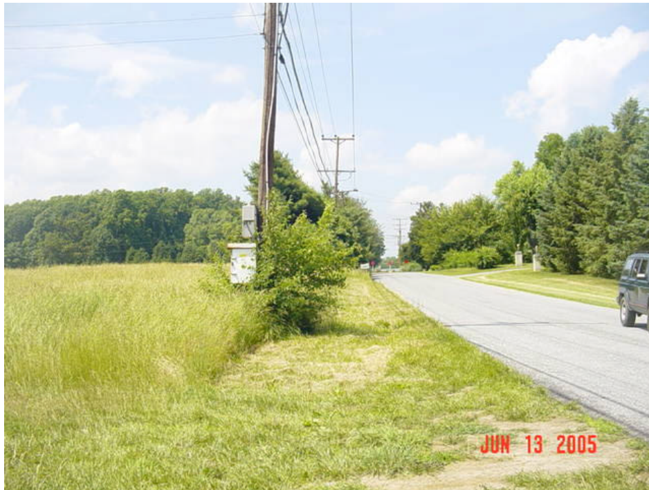
Figure 12 - Impressed Current Rectifier BGE3
