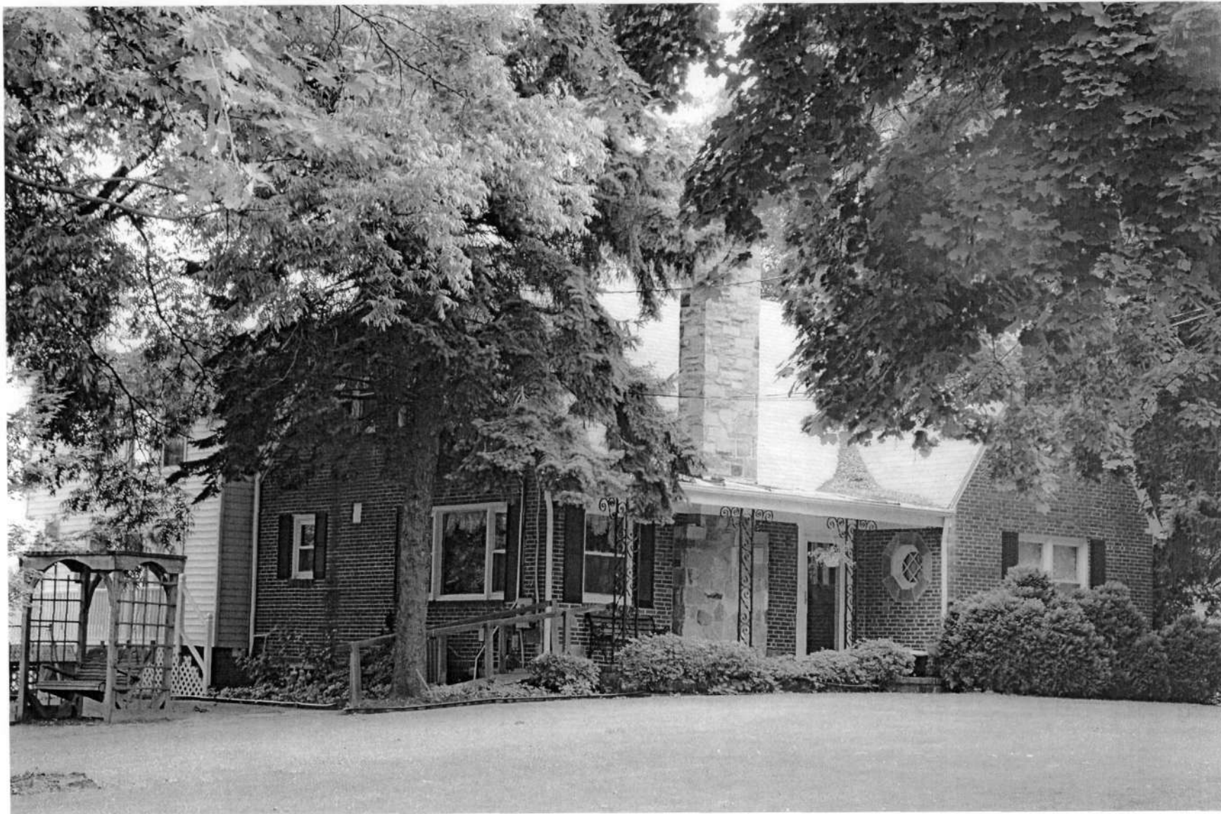
HO-934 8813 Old Frederick Road East & north elevations Ken Short, July 2007 1/1
