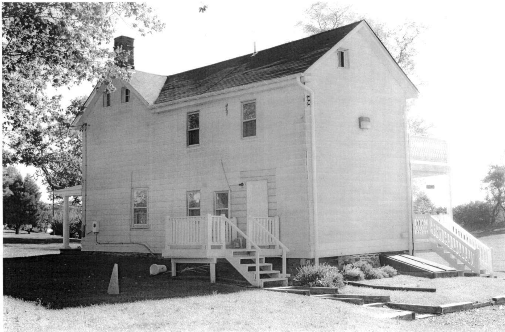
HO-916 "Mount View" Farm 12985 Frederick Road Northwest & southwest elevations Ken Short, October 2006 3/7
