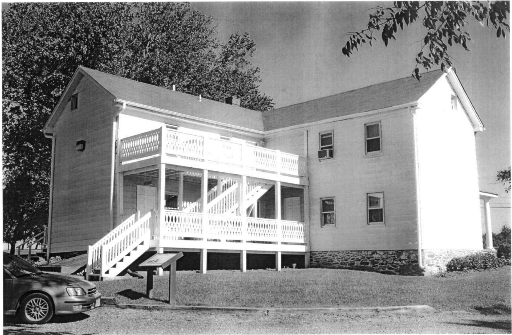
HO-916 "Mount View" Farm 12985 Frederick Road Southwest & southeast elevations Ken Short, October 2006 2/7
