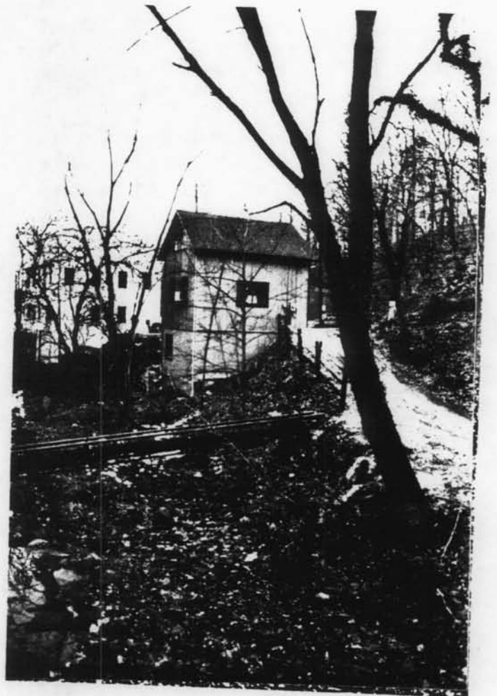
Fig. C-2 Left and rear side elevations after rehabilitation. Left elevation has replicated sliding wooden sash to match what existed originally. On rear, new window installed at basement level; heat pump shown in first floor window; and single window in attic converted to pair unit
